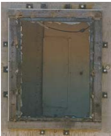
Exterior view of the unprotected window after the test.
